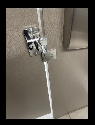
Misaligned doors: A misaligned door is a door that doesn't fit squarely within its frame. This can be due to incorrect installation or damage to the door or frame. Misaligned doors can be difficult to close and may not provide a secure fit, leaving gaps that can be exploited by an intruder.
